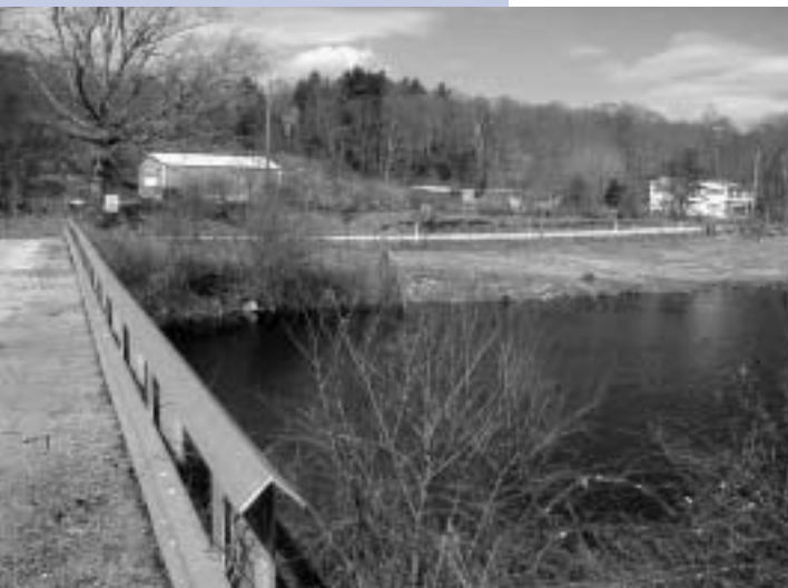
▲ View from the Boom Bridge access
